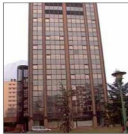
Plaza-Tower, Bozen eg
